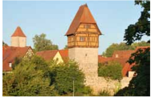
Tower in Dinkelsbuehl (Bauerlinsturm) – Middle Franconia
