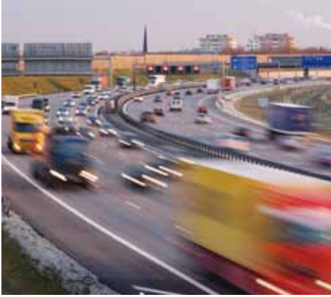
Road infrastructure: Ultra-modern and area-wide
